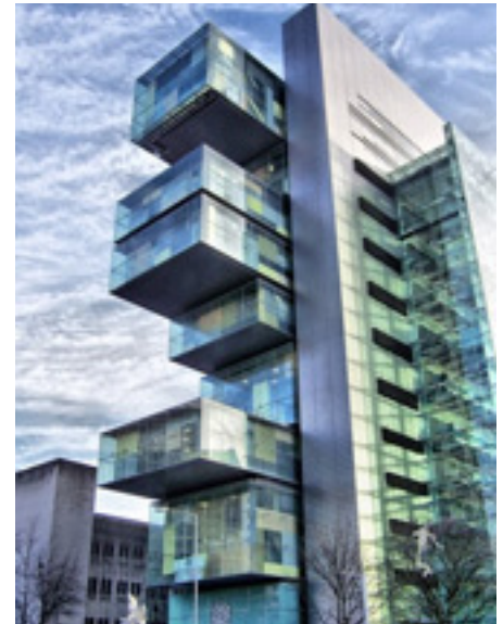
Manchester Civil Justice Center, UK
